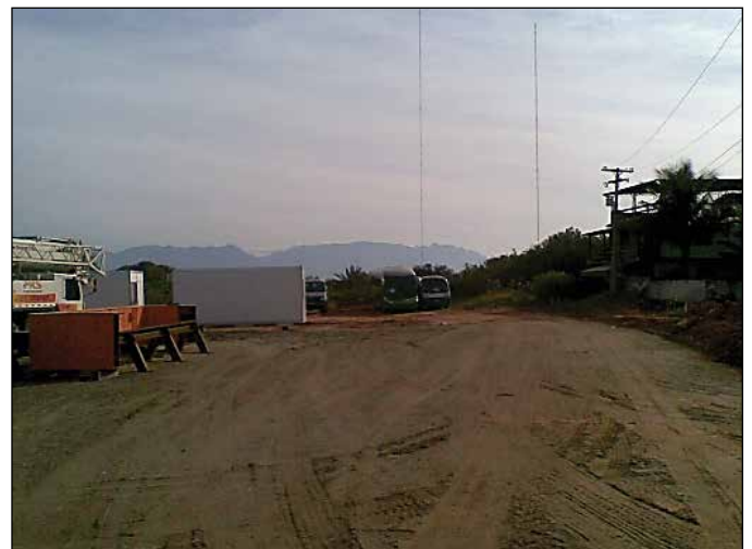
Figure 3 • The antenna towers as seen from the construction site.
